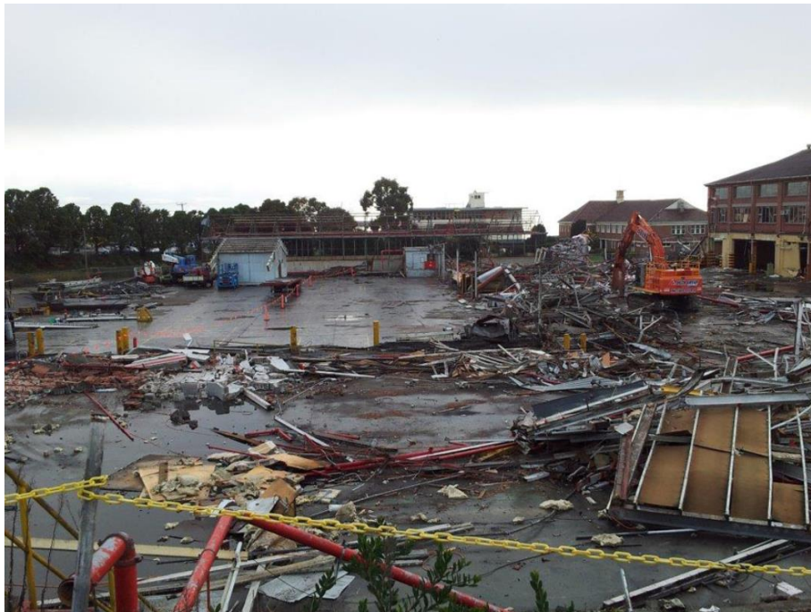
Finishing Room (ground floor) in 2012
